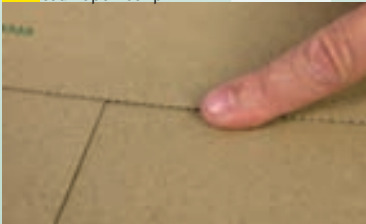
Secure circumferential edge protection
